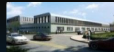
Intelligent network and EMC test room
