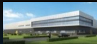
BEV test room
