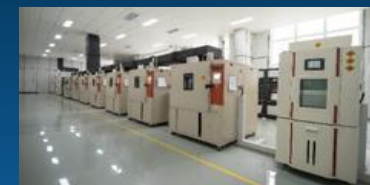
Battery test room
